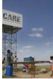
Hoedspruit, Limpopo province: A Roundabout Playpump, a water pump and storage tank at a rural school in the Acornhoek area. The pump is built into the merry-go-round, which, when turned as children play on it, pumps underground water into the tank. Photo: Chris Kirchoff , MediaClubSouthAfrica.com
