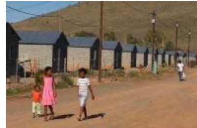
Victoria West, Northern Cape province: New housing with Eskom power installations. Photo: Graeme Williams, MediaClubSouthAfrica.com
