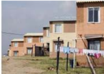
Johannesburg, Gauteng province: Two-storey low-cost walkup housing project in Alexandra township's East Bank. Photo: Chris Kirchoff, MediaClubSouthAfrica.com.
