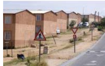
Johannesburg, Gauteng province: Two-storey low-cost walkup housing project in Alexandra township's East Bank. Photo: Chris Kirchoff, MediaClubSouthAfrica.com.
