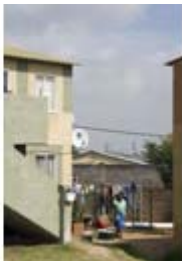
Johannesburg, Gauteng province: Two-storey low-cost walkup housing project in Alexandra township's East Bank. Photo: Chris Kirchoff, MediaClubSouthAfrica.com.
