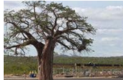
Limpopo province: A new construction to monitor transport from Zimbabwe is built next to a baobab tree on the N1 freeway, north of Musina. Photo: Graeme Williams, MediaClubSouthAfrica.com
