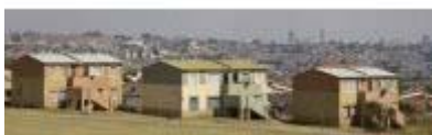
Johannesburg, Gauteng province: Two-storey low-cost walkup housing project in Alexandra township's East Bank. Photo: Chris Kirchoff, MediaClubSouthAfrica.com.
