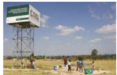
Hoedspruit, Limpopo province: A Roundabout Playpump, a water pump and storage tank at a rural school in the Acornhoek area. The pump is built into the merry-go-round, which, when turned as the children play on it, pumps underground water into the tank.
