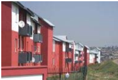
Johannesburg, Gauteng province: Low-cost housing project adjacent to Freedom Square in Kliptown, Soweto. Photo: Chris Kirchoff, MediaClubSouthAfrica.com.
